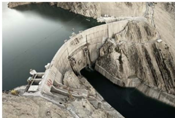
Fig 4 Karun 3 dam and its reservoir and appurtenant
