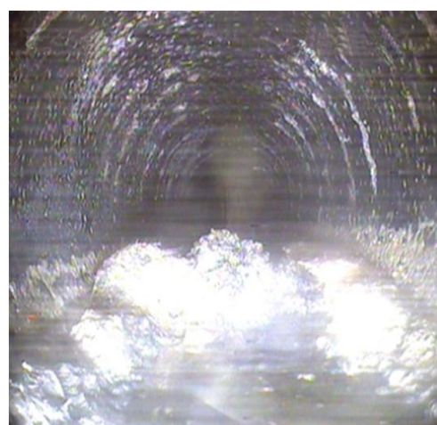
Fig. 13 Facing robot with large deposit during sewer pipe inspection
