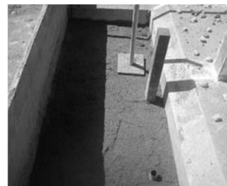
Fig.4. Compaction hammer and sampling can
